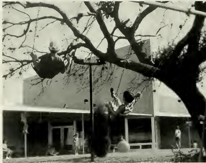
Child Care Center, Sarasota Memorial Hospital, Carl Abbott FAIA. Large windows admit natural light, allow visual surveillance for safety. Tall central space allows hot air to rise. Windows and doors open for cross-ventilation. Photograph: Cooper Abbott
